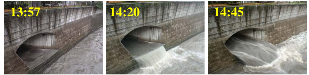
Fig. 1 Combined sewer overflow at the Edogawabashi Brg. of Kanda River on 8 th Sep. 2010
